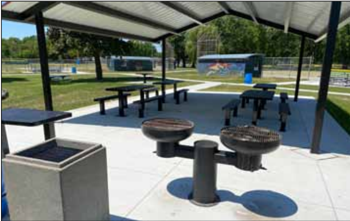
The new shelter has grills, a prep table, and picnic tables.
